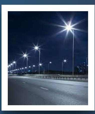
Highway street light with 9-meter pole, 250W LED (Syska), Day/Night Sensor, Separate MCB and earthing for each pole.
